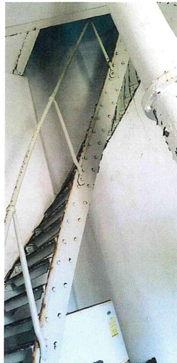
Pic. 7 Ladder from ground to 1 st floor
