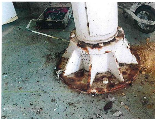
Pic. 3 Vertical pipe bolted to ground floor slab
