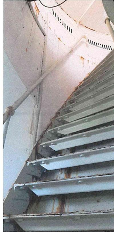
Pic. 9 Ladder from 2 nd floor to 3 rd floor.
