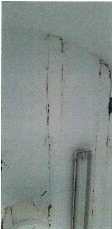
Pic. 6. Soffit of 1 st and 2 nd floor slabs.
