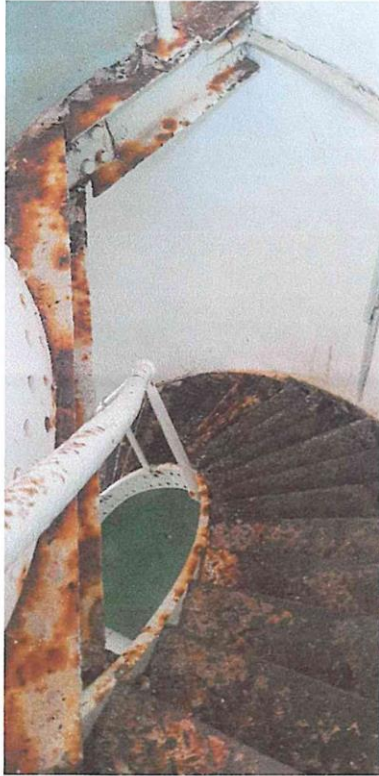
Pic 8. Ladder from 1 st floor to 2 nd floor.
