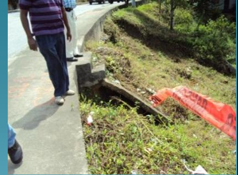
L56-St. Croix Road LP#85- 86 RHS
