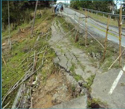
L57-St. Croix Road LP#87-88 RHS
