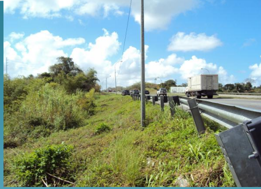
L63 – SHH Macaulay Overpass
